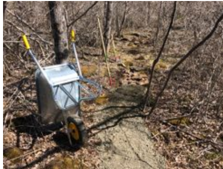
Volunteers are adding rock and gravel to make a smoother drier trail surface in some of the trail’s rougher sections.
