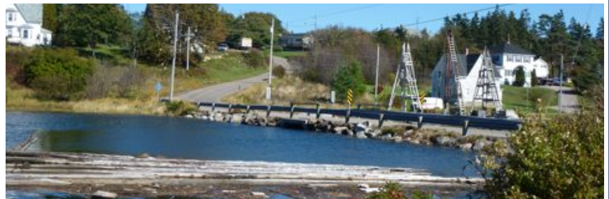
Not much room left under the bridge!
