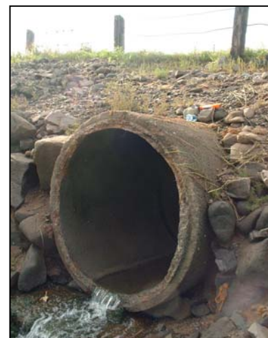
Figure 12. Downstream end of culvert at low tide.
