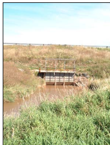
Figure 4. Wellington Dyke and Aboiteau, NS. Site KCMB10A
