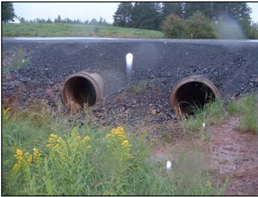
Figure 20. Downstream view showing culverts placed above the base of the channel. The background shows a definite elevation rise and a mix of agriculture and woodland upstream.
