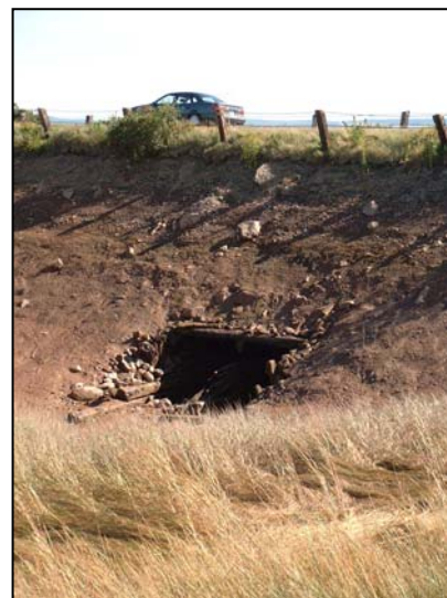
Figure 14. Upstream view of crossing at low tide
