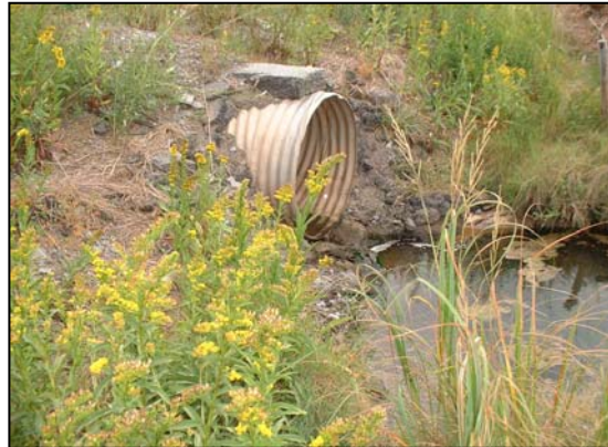
Figure 22. Upstream view of culvert
