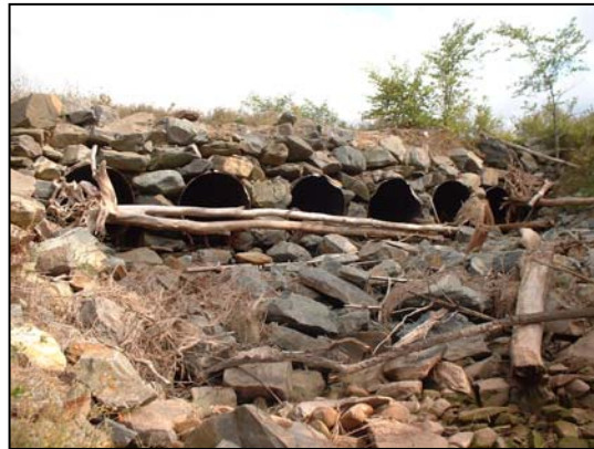
Figure 11. Upstream view of the six overflow aboiteaux.
