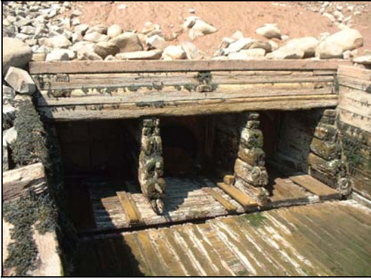
Figure 8. Downstream view of crossing
