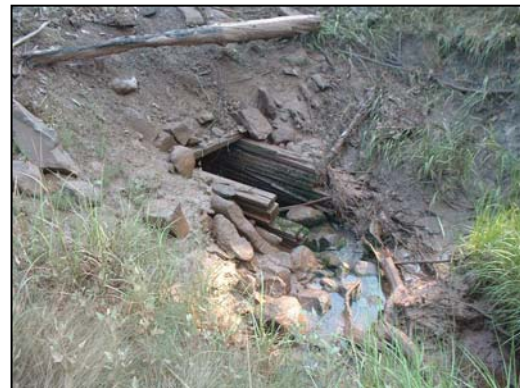
Figure 23. Upstream of crossing at low tide
