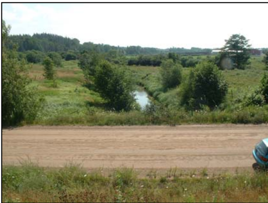
Figure 36. Photo taken from top of the dyke looking upstream. The dirt road and fallow upstream lands are visible.
