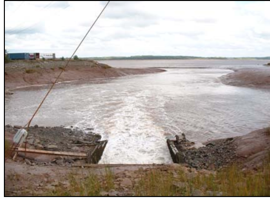
Figure 9. The extremely turbulent outflow through the comparatively small culvert.
