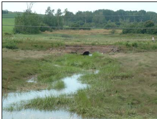
Figure 13. Upstream of crossing showing wetland area and driveway culvert.
