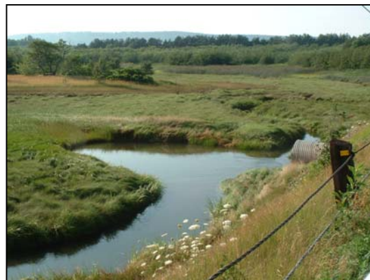
Figure 17. Upstream of crossing, large scour pool, stream branches off in two directions (low tide).
