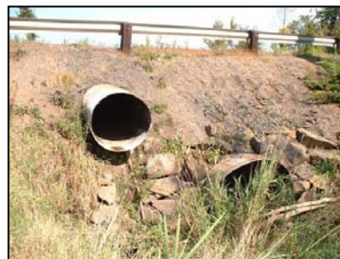
Figure 2. Hanging culvert within a causeway, Kentville, NS. Site KCMB7C
