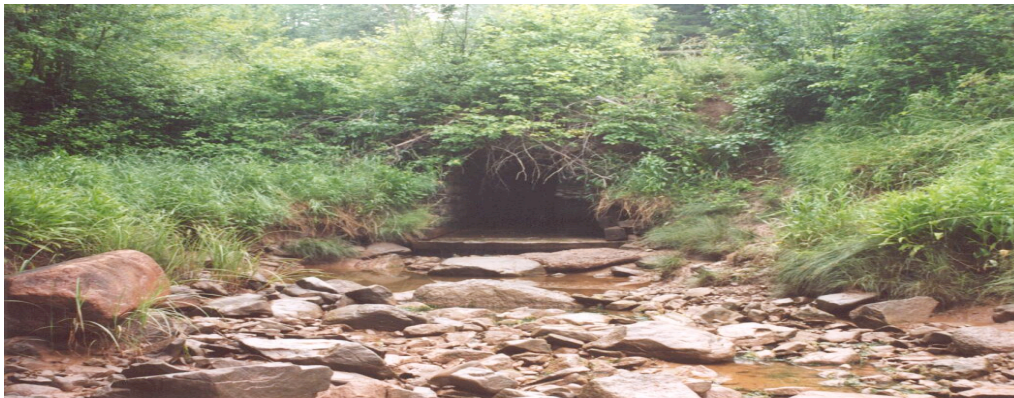
Figure 26. Downstream view of a wooden box culvert at site SHIC (Princeport).
