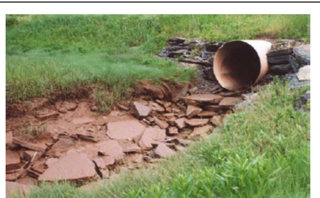
Figure 2. Photograph of a culvert situated at site SH2C.
