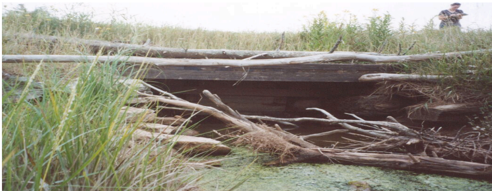
Figure 25. Downstream view of an old wooden aboiteau at site CBSS14A (Black Rock).
