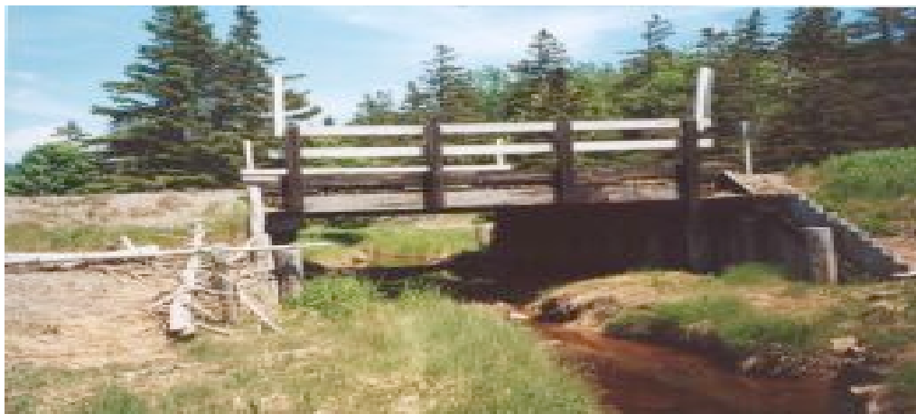
Figure 31. Downstream view of a bridge at site CBNS13B (Carrs Brook).
