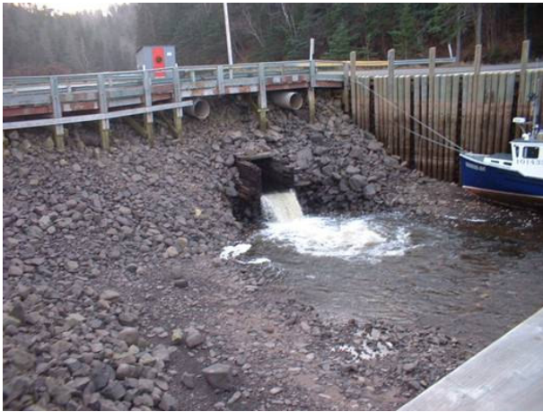
Figure 1. Downstream view of crossing
