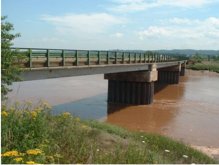
Figure 1. Cornwallis River bridge in Port Williams.
