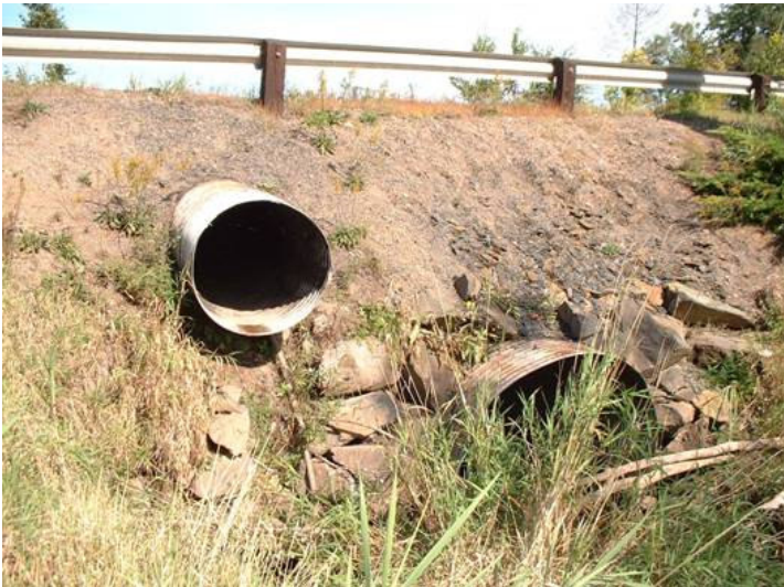
Figure 1. The culvert and drainage pipe.
