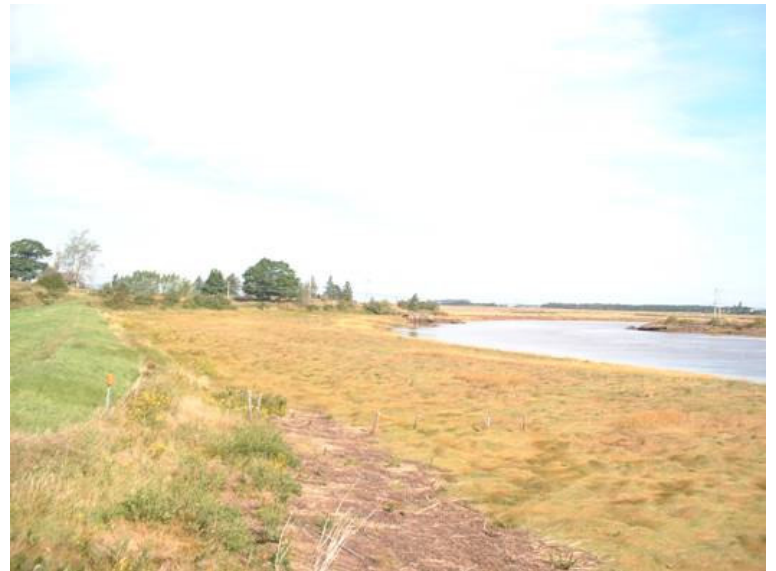
Figure 2. Upstream showing dykes along the river edge.
