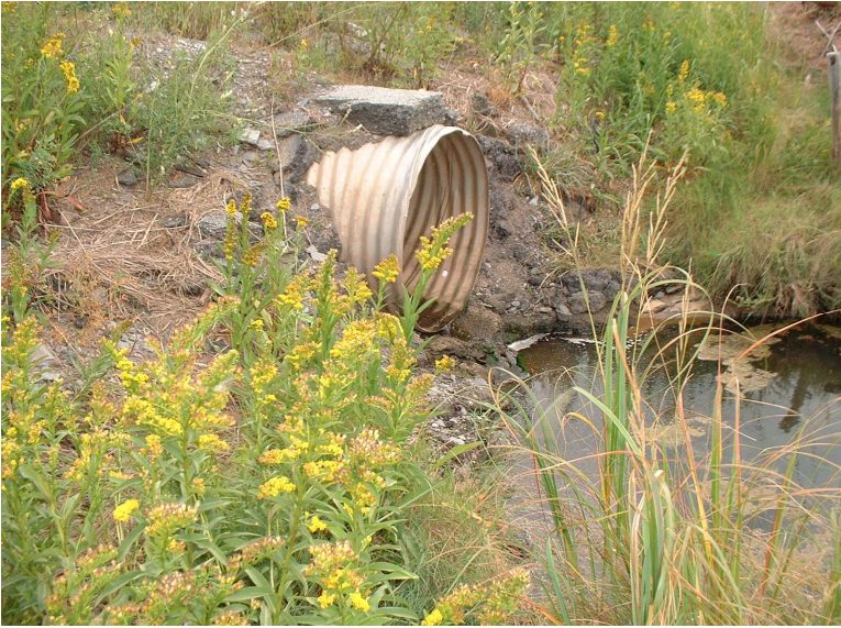
Figure 1. Upstream of culvert.
