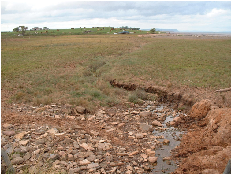
Figure 2. Downstream of culvert.
