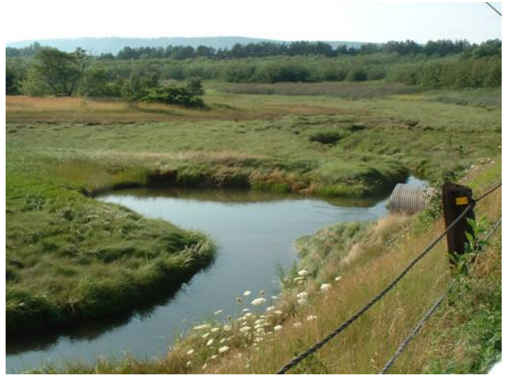
Figure 1. Upstream of crossing, large scour pool, stream branches off in two directions.
