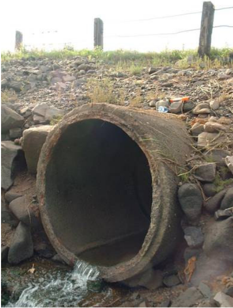
Figure 1. Downstream end of culvert at low tide.
