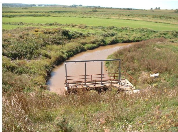
Figure 2. Upstream farmland being protected by the dyke and aboiteau. The creek is fresh water.
