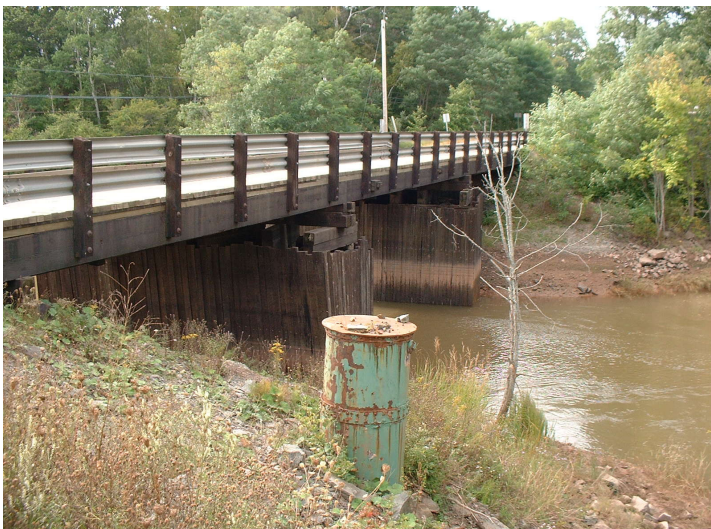
Figure 1. Upstream photo of the bridge.
