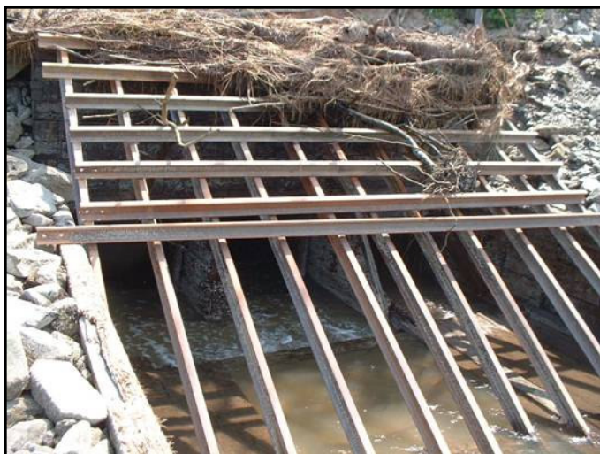
Figure 5: replacement or removal of broken gate would reduce the accumulation of debris
