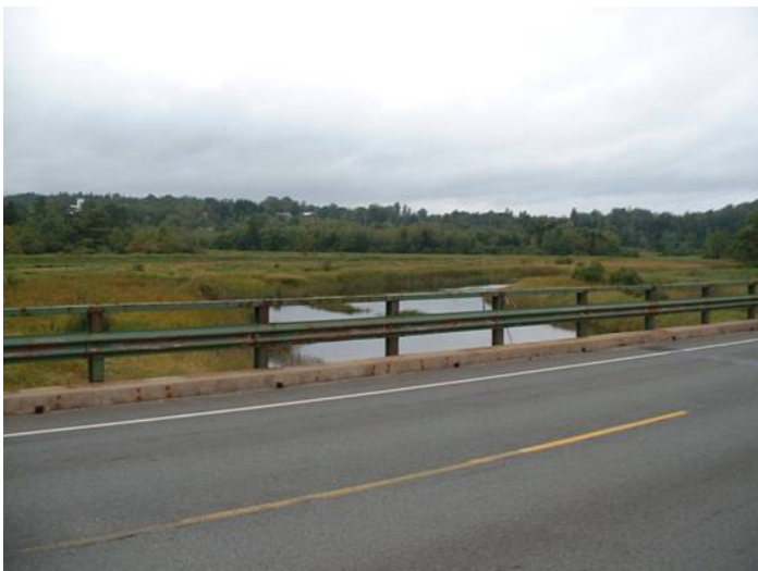
Figure 3. Looking upstream from the bridge.
