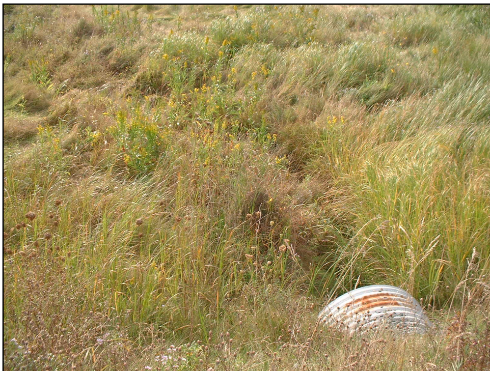
Figure 1: Downstream end of culvert and wetland surface.
