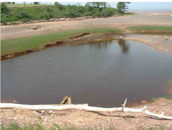
Figure 5. Downstream scour pool
