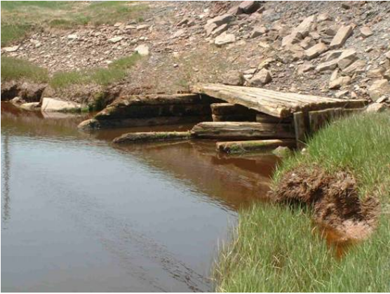
Figure 1. Upstream view of crossing
