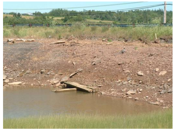
Figure 4. Downstream view of crossing
