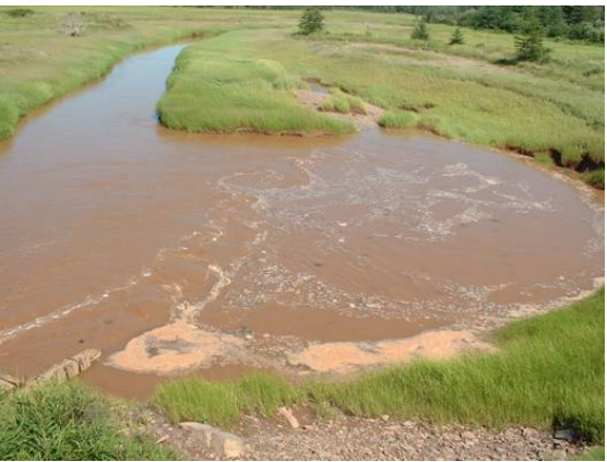
Figure 3. Upstream scour pool
