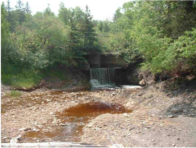
Figure 1. Downstream view of crossing
