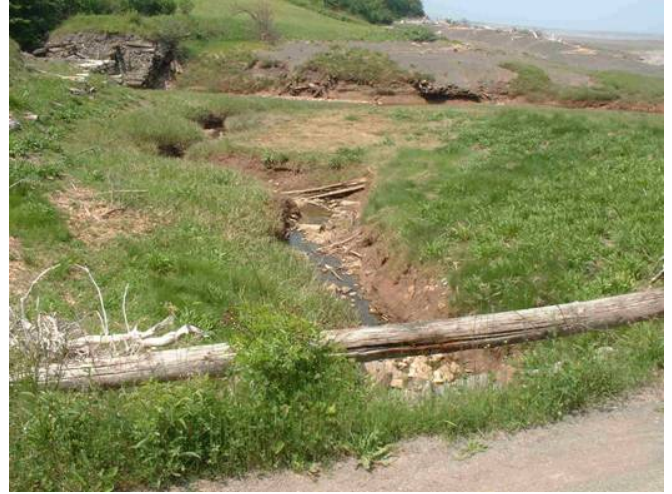
Figure 2. Downstream of crossing
