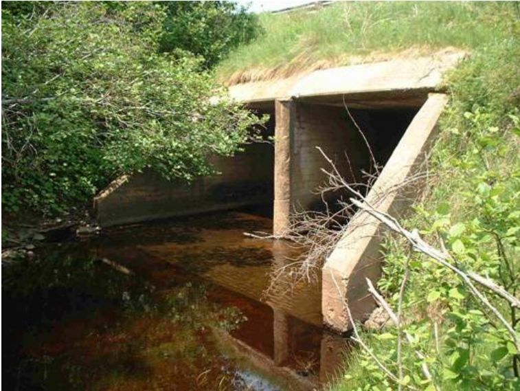
Figure 5. Upstream view of crossing
