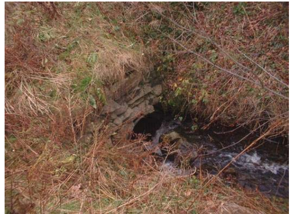
Figure 2. Upstream view of crossing.
