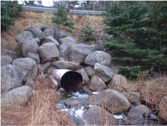
Figure 1. Downstream view of culvert Area is wooded
