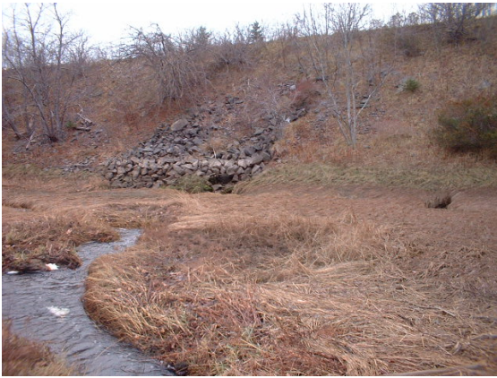
Figure 1. Upstream view of crossing
