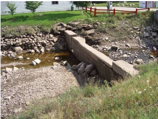
Figure 2. Dam just downstream of crossing
