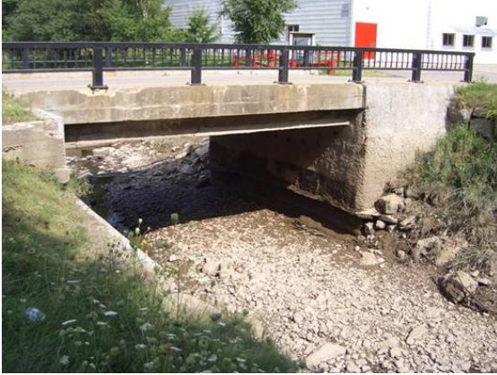
Figure 1. Downstream view of crossing
