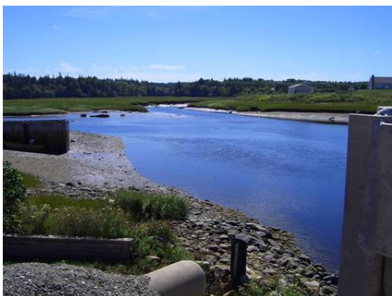
Figure 3. Upstream of crossing, river divides just upstream of crossing. Old structure is visible in picture
