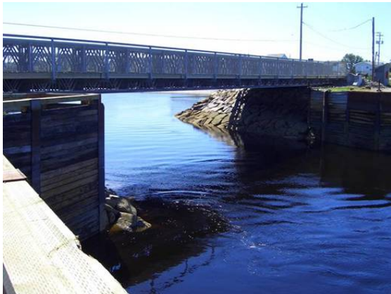
Figure 1. Downstream view of crossing
