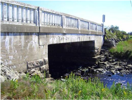
Figure 1. Downstream view of crossing
