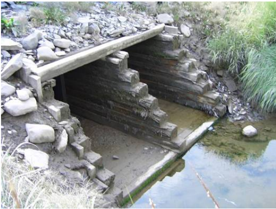
Figure 1. Downstream view of crossing branches from main channel of Bear River
