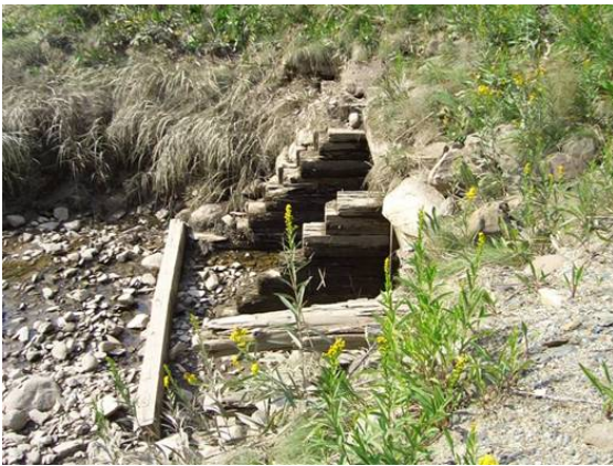
Figure 3. Upstream view of crossing, some debris around opening
