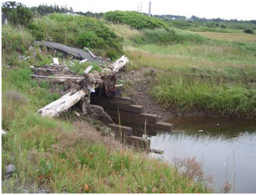
Figure 1. Downstream view of culvert
