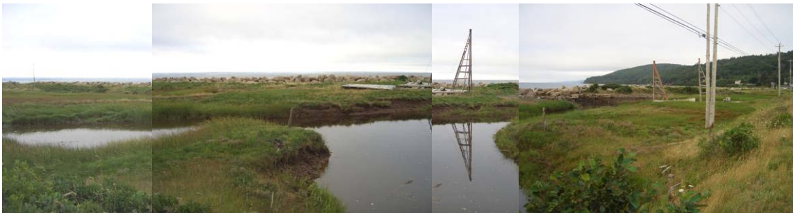
Figure 3. Downstream of crossing showing scour pool to the left (east) of the crossing. Main channel flows out through the seawall.
