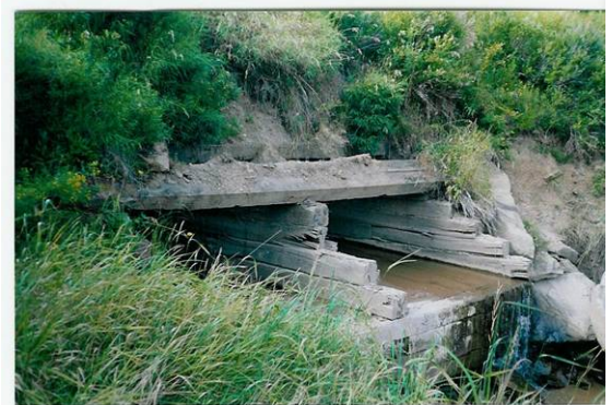
Figure 4. Close up of the old, double chambered, wooden culvert.
