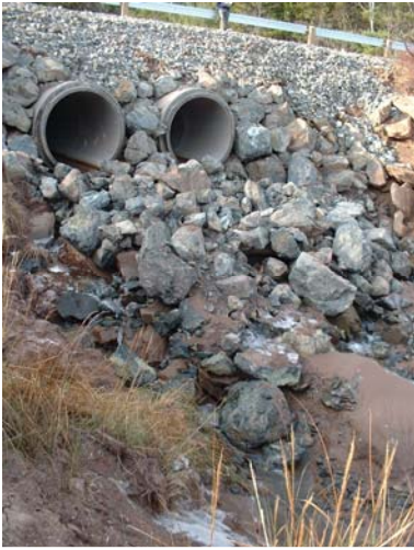
Figure 1. The downstream view of the new culverts.
