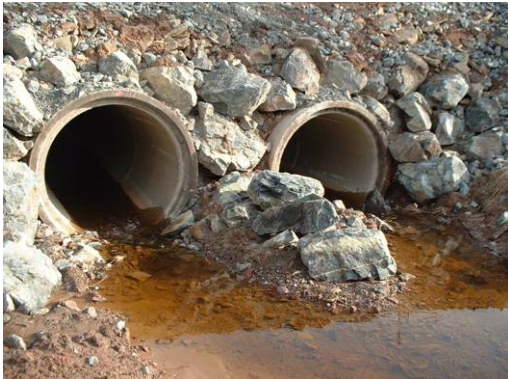
Figure 3. Upstream of the new culverts.
