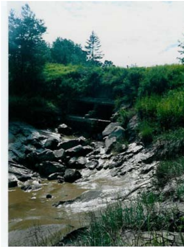
Figure 2. The downstream view of the old culverts
