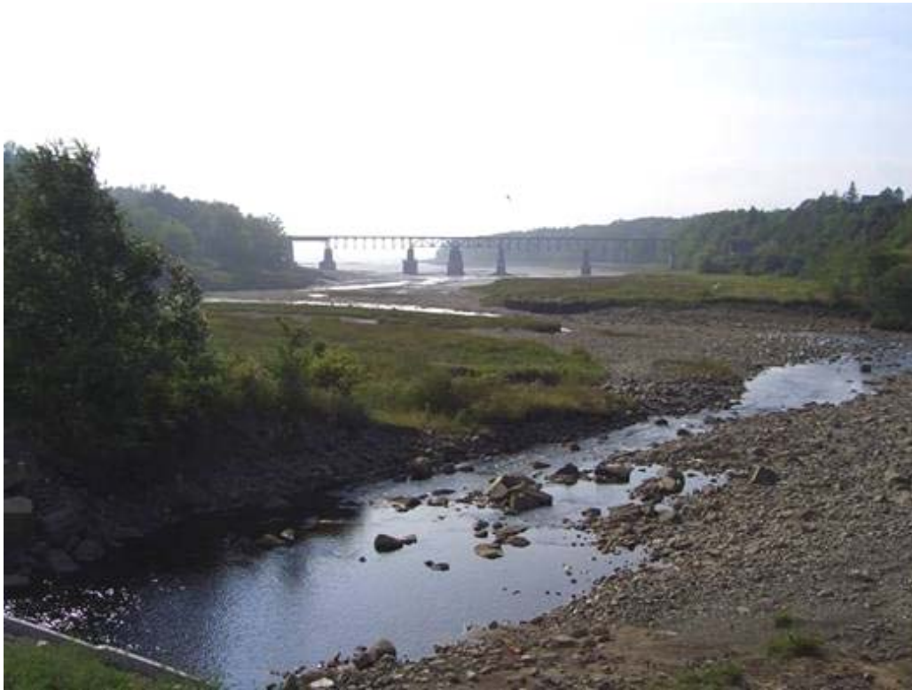
Figure 2. Downstream of crossing
