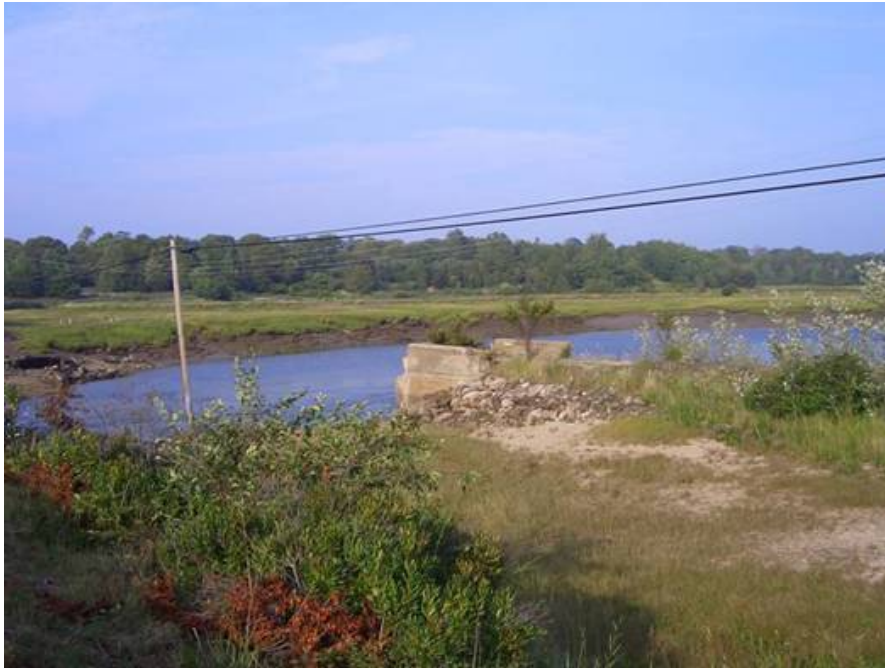
Figure 2. Upstream remnants of old Crossing.
