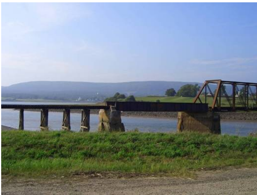
Figure 3. View of downstream and rail bridge
