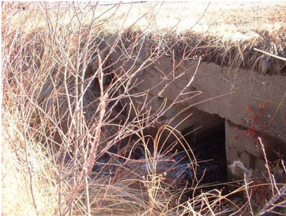
Figure 3. Upstream view of crossing
