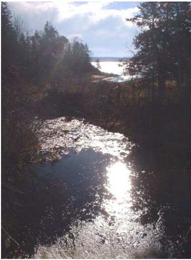
Figure 2. Downstream of culvert
