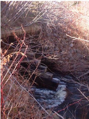
Figure 3. Upstream view of culvert.
