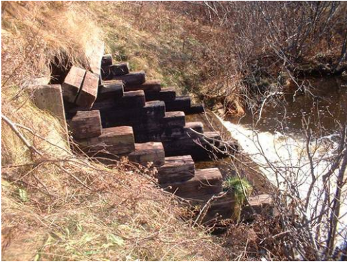
Figure 1. Downstream view of crossing.
