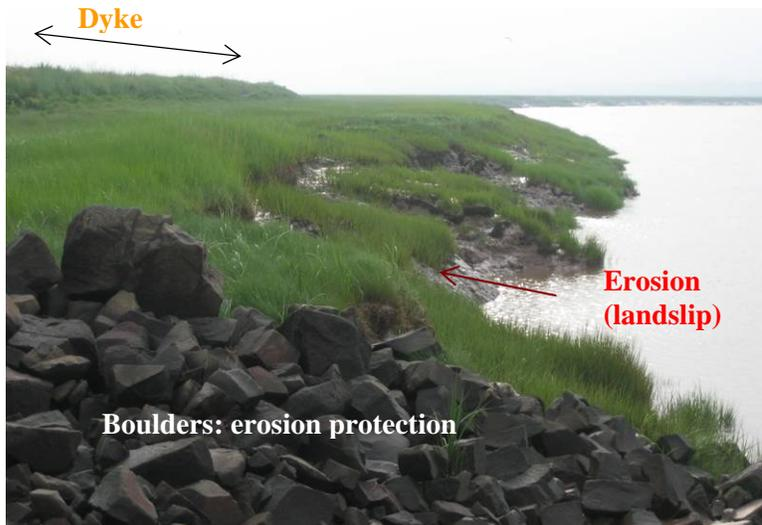
**Photo 1.** Boulders on the left bank that protect against erosion, near the old dyke. Looking eastward.
